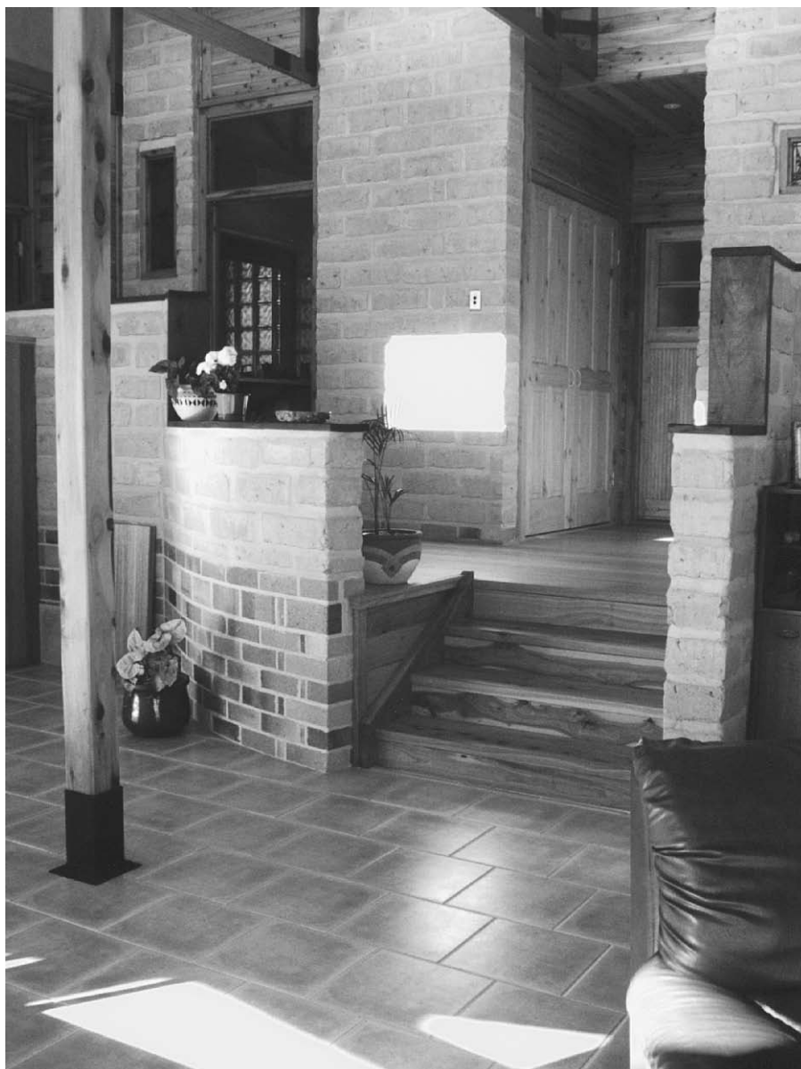
Curving half walls enhance the change in levels from heat slab to timber floored rear.
