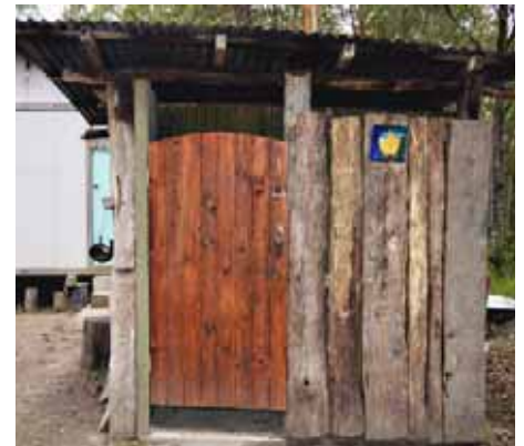
Clockwise from left: Door handles hand crafted from tree branches; recycled corrugated roof sheeting has been used as internal lining; doors are of recycled boards; volunteer humour – a Holden headlamp 'shines' from the concrete slab; on-site timber was used for external cladding – vertically and horizontally.
