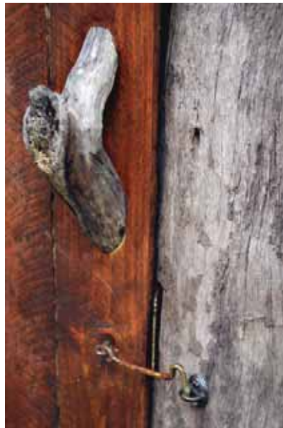
Clockwise from left: Door handles hand crafted from tree branches; recycled corrugated roof sheeting has been used as internal lining; doors are of recycled boards; volunteer humour – a Holden headlamp 'shines' from the concrete slab; on-site timber was used for external cladding – vertically and horizontally.
