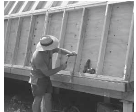
Fixing the cyclone straps to base.
