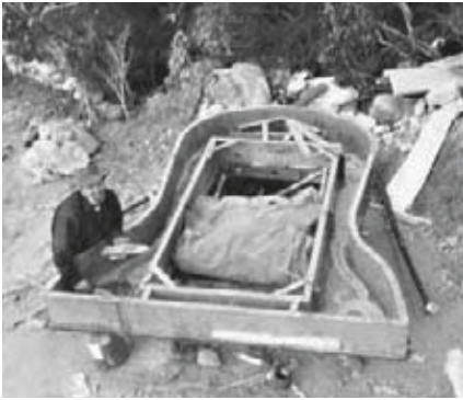
L-R: Trailer-mounted mould for the concrete arches; cypress pine lining jigsaw; roof framing.
