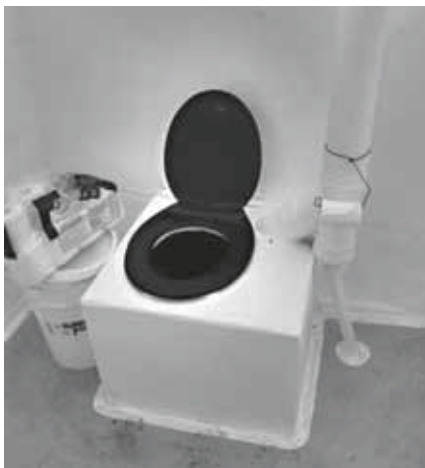
Left: Seat is usually left down to help create a seal. The condensation tube returns moisture to the pit. Bucket contains chaff. Top right: Removing the access panel (left pit) exposes the baffle & aeration pipes (right pit). Rest: the toilet at various stages of construction.
